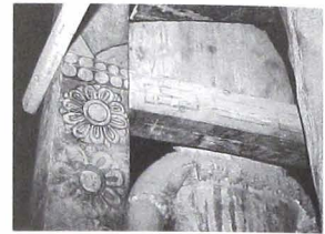
Fig. 212. Ladder-like scaffolding for the sculptures painted with simple geometrical and flower motifs Main Temple, passage between the back of the temple (Ambulatory and Cella) and the Assembly Hall, back of sculpture IV
